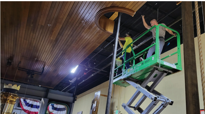
Chase and Quinn with Clinton Electric installing new track lighting.
